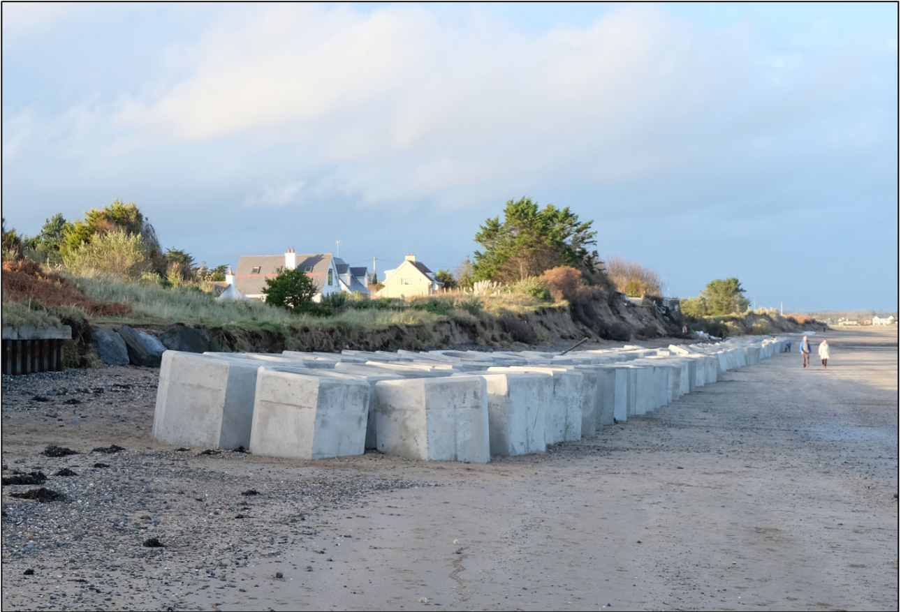
Figure 1.4: General layout of the temporary interim coastal protection measures along the Burrow – Dec 2018
