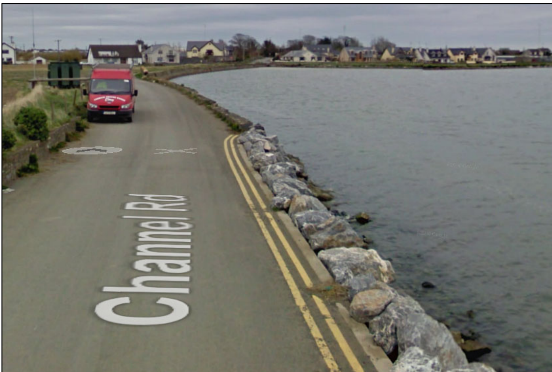
Figure 1.14: Low crest level of the existing rock revetment at the western extent of Channel road (© Google Earth)
