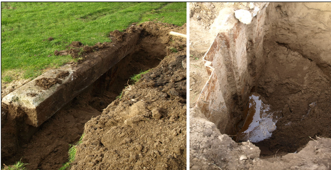
Figure 1.7: Buried sheet piling in front of Brook pub – July 2019
