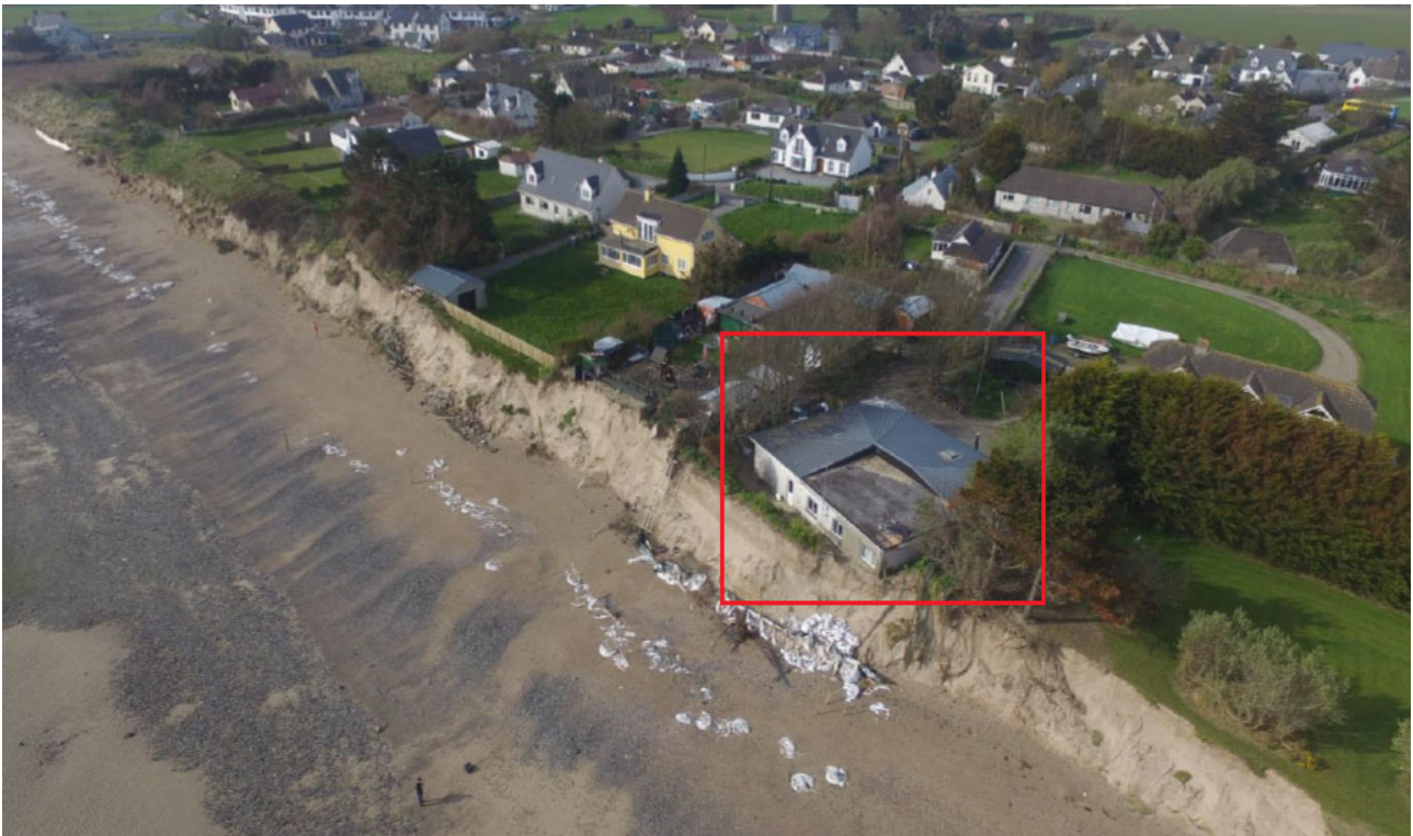
Figure 2.4: Aerial view of the residential property (inside of red box) that was demolished following the extreme winter period of 2018
