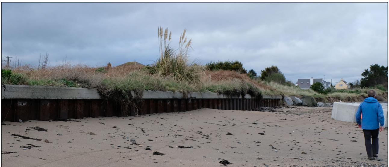
Figure 1.6: Exposed sheet piling along the southern section of the Burrow
